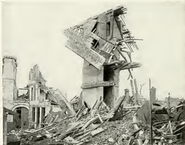
LA BASSÉE. CONCRETE OBSERVATION-POST BUILT BY THE GERMANS INSIDE A HOUSE WHICH, LATER, COLLAPSED
