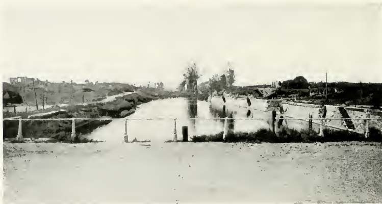
ENTRANCE TO YPRES. YPRES CANAL, AT BOESINGHE, SEEN FROM RUE DE DIXMUDE, YPRES
