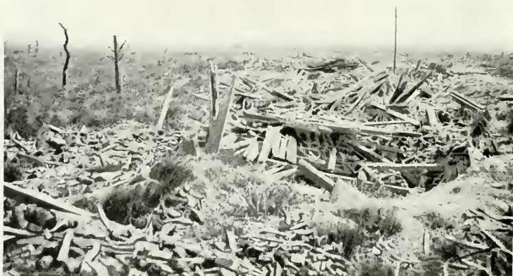
WHAT WAS ONCE PASSCHENDAELE. THE CHURCH WAS ON THE HILLOCK IN THE BACKGROUND
