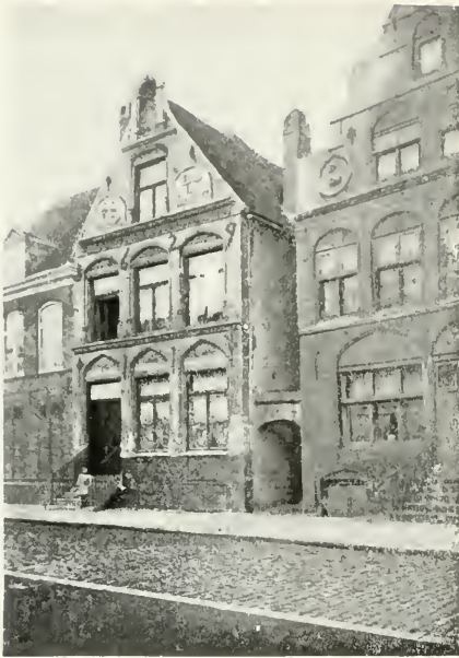
THE MAISON DES BATELIERS (1629) Completely destroyed. Note the two emblem- atical ships on the façade. (Photo, Antony, Ypres.)
