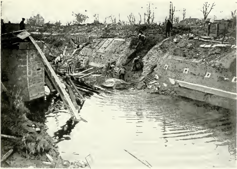
DESTROYED BRIDGE ACROSS THE BASSÉE
