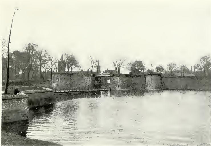
THE RAMPARTS, LILLE GATE AND ST. PETER'S CHURCH
