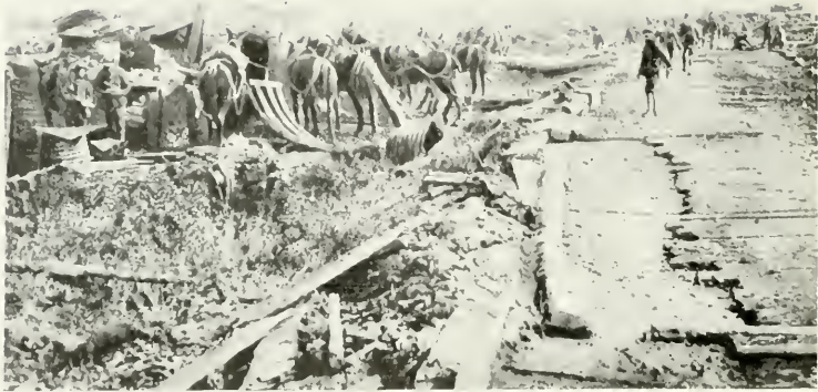
DURING THE WINTER MONTHS LOG-ROADS WERE NECESSARY FOR THE LORRIES AND ARTILLERY, AND EVEN THESE SANK IN THE BOTTOMLESS MUD
