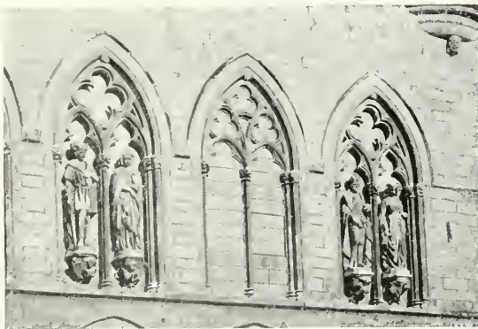
THE WINDOWS OF THE FIRST STOREY OF THE CLOTH HALL Every alternate window was blind, and was ornamented with statues of the Counts of Flanders or other notable persons of the city (photo, Antony, Ypres).
