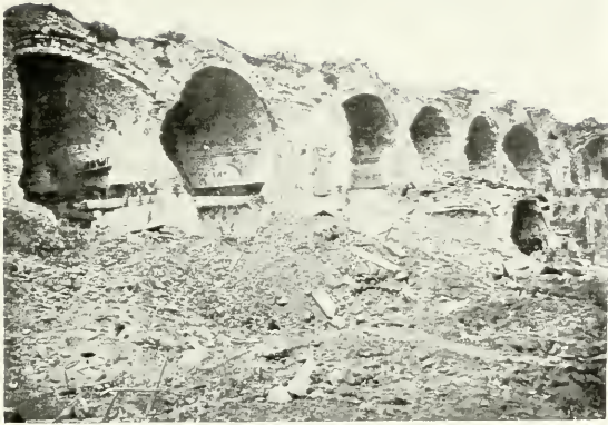
VAULTING OF THE OLD FRENCH BARRACKS
