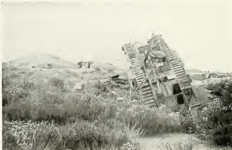
LANGEMARCK, WITH DESTROYED TANK. THE MOUND IN THE MIDDLE DISTANCE IS ALL THAT REMAINS OF THE CHURCH
