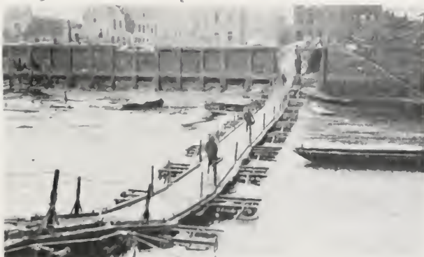
TEMPORARY FOOT-BRIDGE ACROSS THE YSER AT NIEUPORT.
