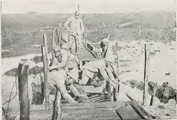
BUILDING A TEMPORARY BRIDGE.
