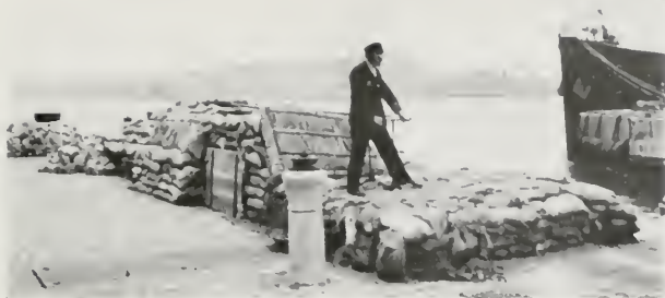
PROTECTING THE MECHANISM OF THE LOCKS FROM THE SHILLS.
