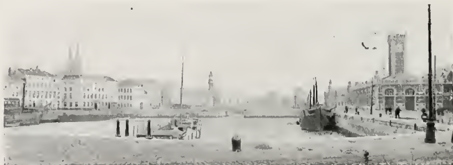
DOCK NO. 2, CHURCH OF ST. PETER AND PAUL (left) and the STATION (right).
