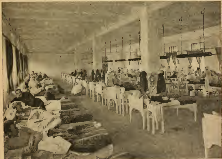
A VIEW OF ONE OF THE WARDS
