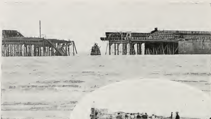
The open-work portion of the Mole destroyed by the British submarine, (Lieut. Sandford). Inset: temporary bridge built by the Germans and destroyed by them before their retreat.
