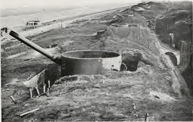
GENERAL VIEW OF THE AACHEN BATTERY ( north-east of Middelkerke-Bains ).
