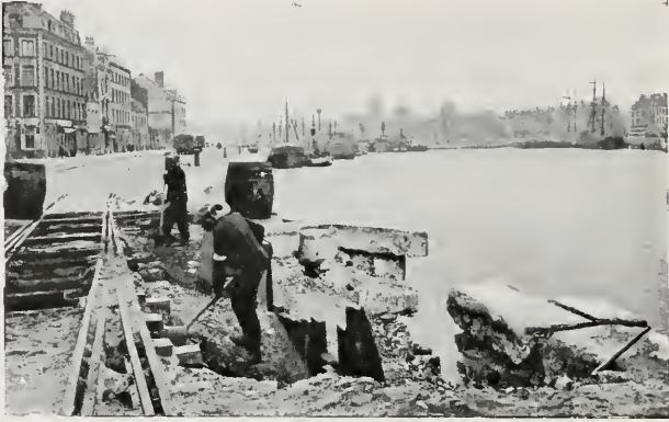
QUAI DE LA CITADELLE STRUCK BY A 15IN. SHELL.
