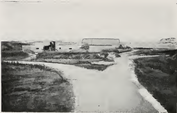
NAPOLÉON FORT, AND THE ROAD LEADING TO THE HINDENBURG BATTERY (on the left).
