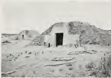
CONCRETE GUN SHELTER, 100 yards east of Coxyde-Bains.
